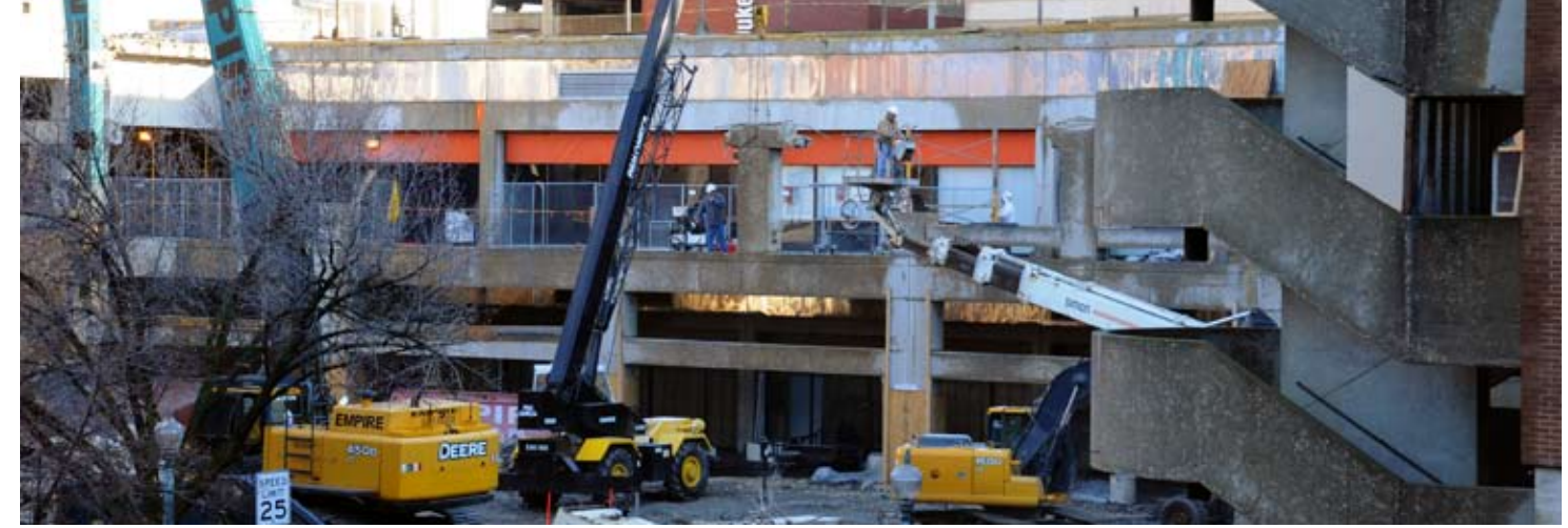
Demolition underway at Lancaster Square.
