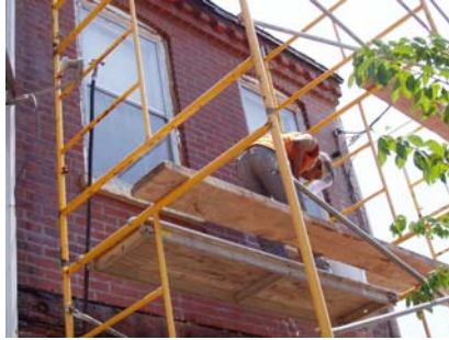
Removing formstone to expose brick
